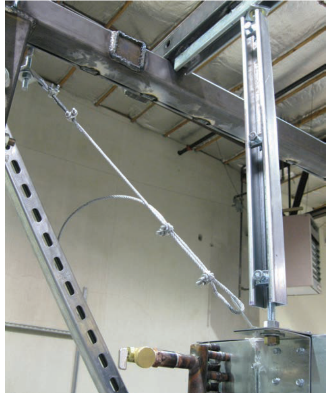
FIG. 6 - UNISTRUT USED TO STRENGTHEN THE ROD
