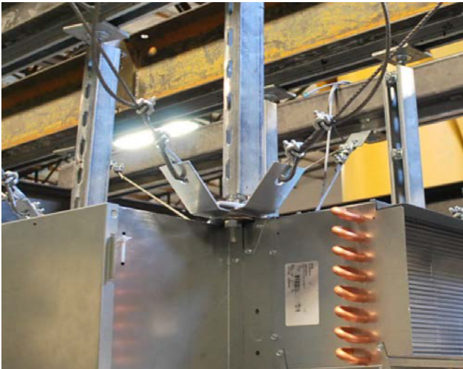
FIG. 7 - OVERLAPPED FLAT AND 45° BRACKETS
