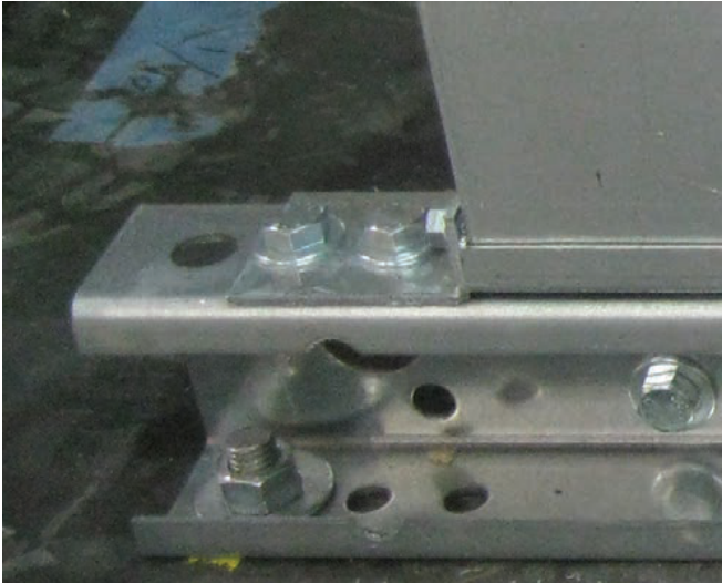
FIG. 10 - BOLT AT EACH BASE-RAIL CORNER
