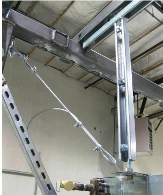
FIG. 8 - UNISTRUT USED TO STRENGTHEN THE ROD
