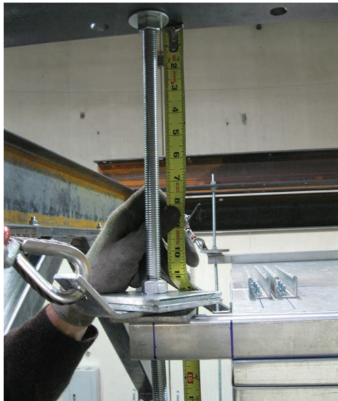
FIG. 4 - RECOMMENDED LENGTH OF THREADED ROD
