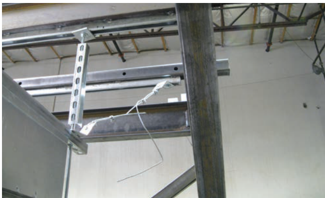
FIG. 3 - LATERAL SUPPORT COMPONENTS FOR SBHD 08-20
