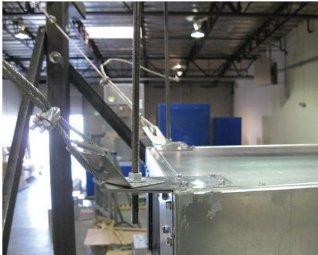
FIG. 5 - OVERLAPPED FLAT, 90° AND 45° BRACKETS
